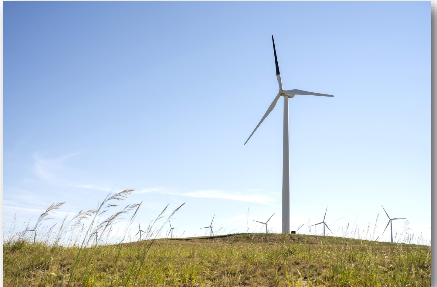
Wind turbine blade painted black at a wind farm near Glenrock, Wyoming operated by PacifiCorp. Credit: PacifiCorp.
